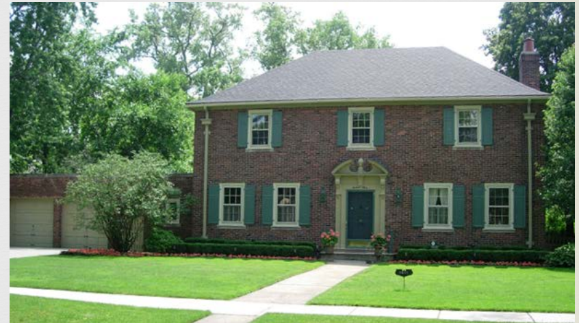
1611 Lincolnshire The Moritz Kahn House, 1935
